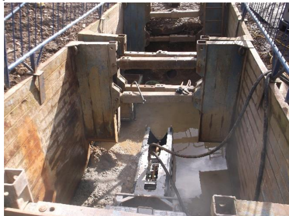
The pipe-bursting power hammer, going underground
