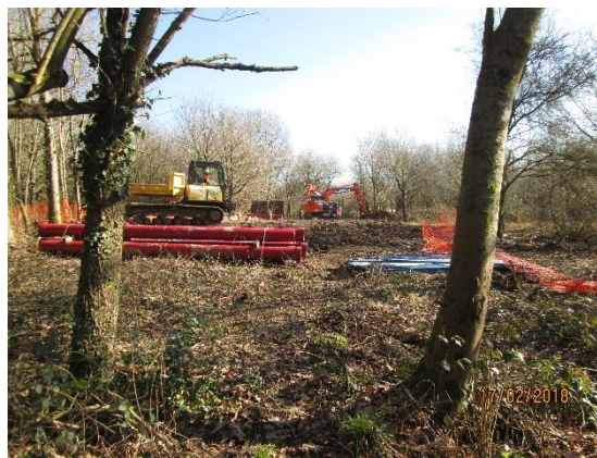
Replacing the pipe across the Park
