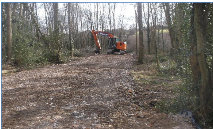
The temporary roadway
